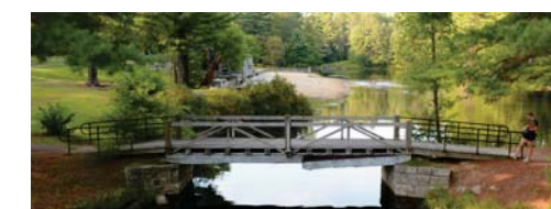
Footbridge over Catamount Pond.
